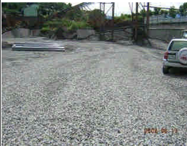
C.堆置區鋪設粗級配
