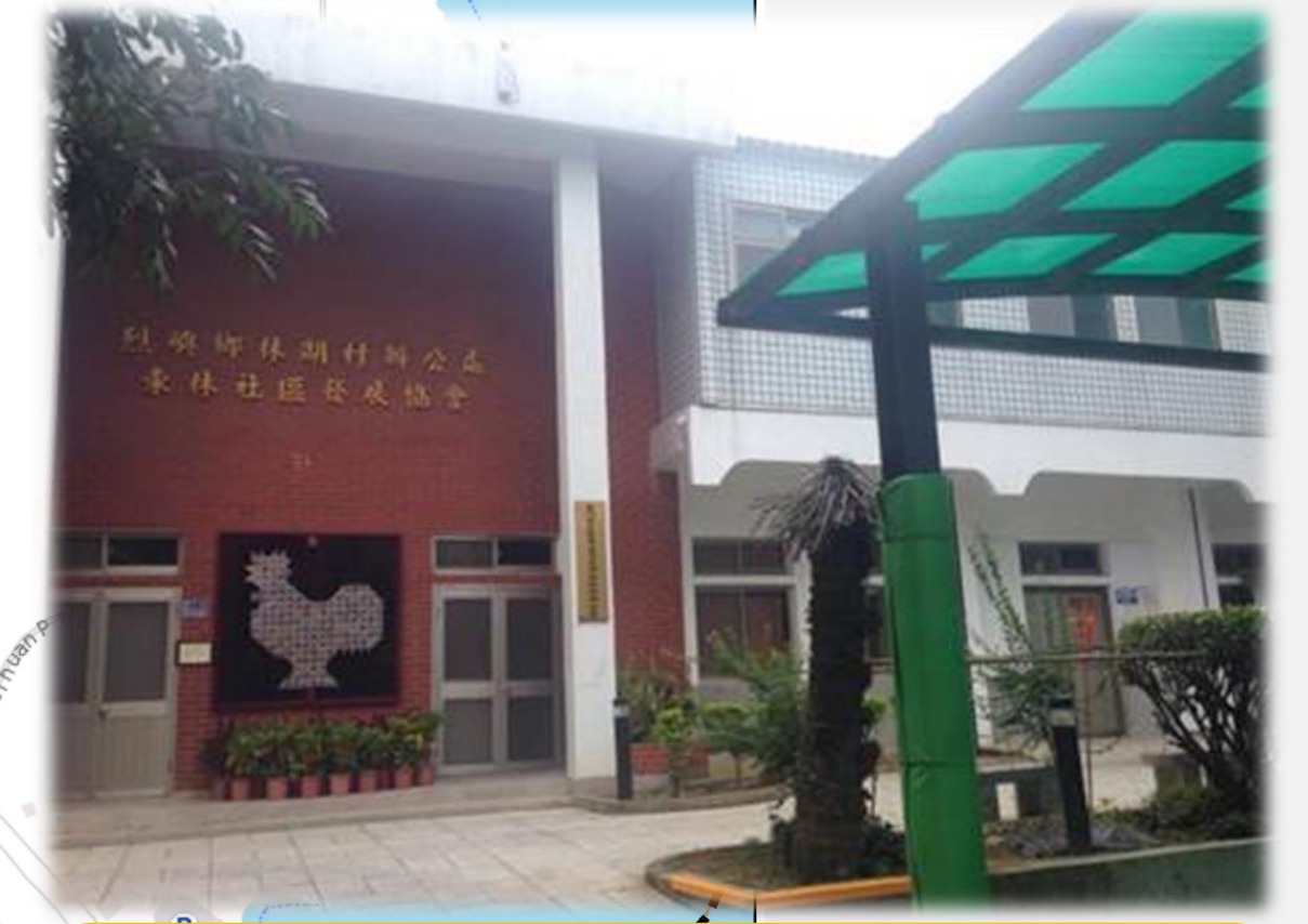
Xikou Village Office Shelter for Flood and Earthquake
