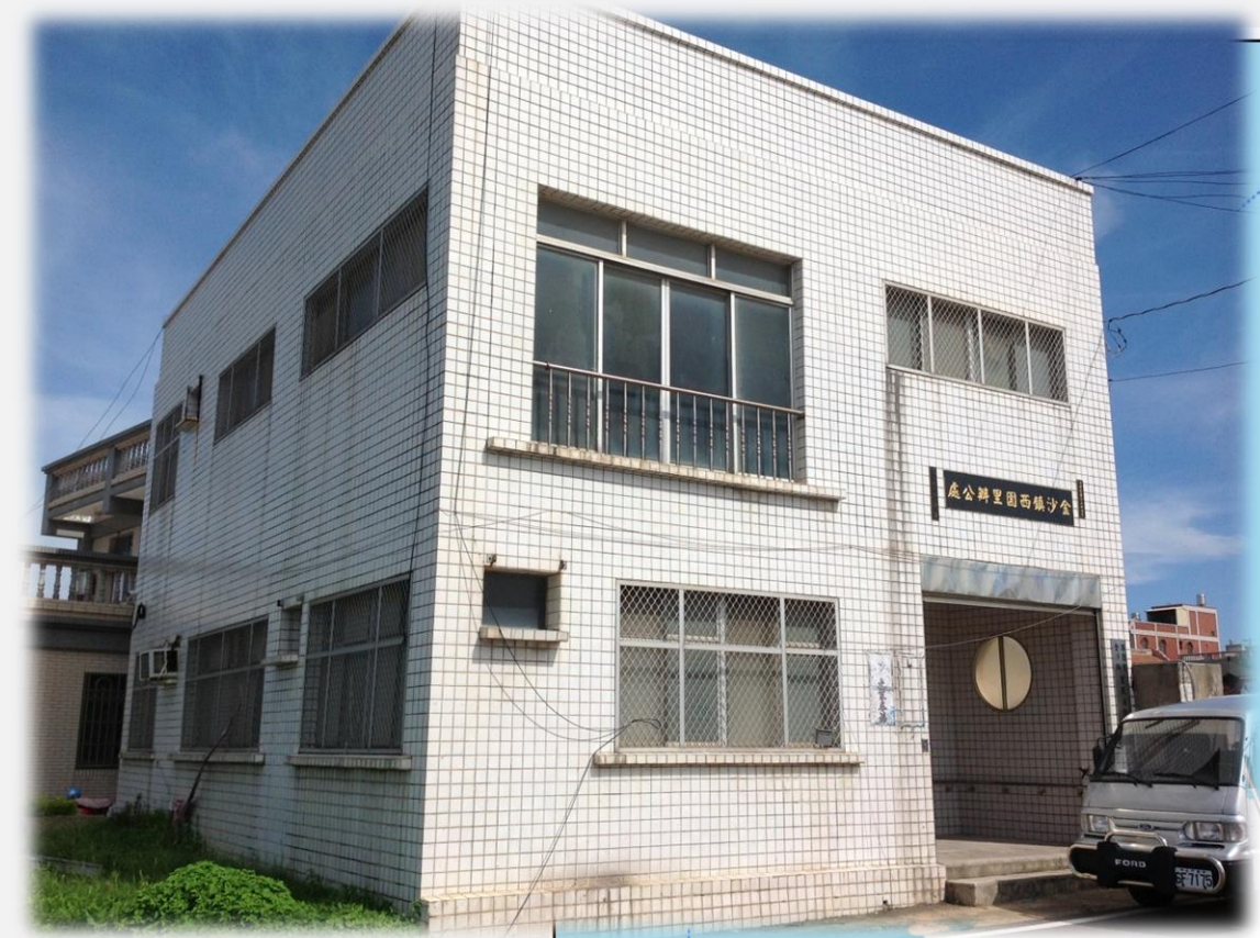
Xiyuan Village Office Shelter for Flood
