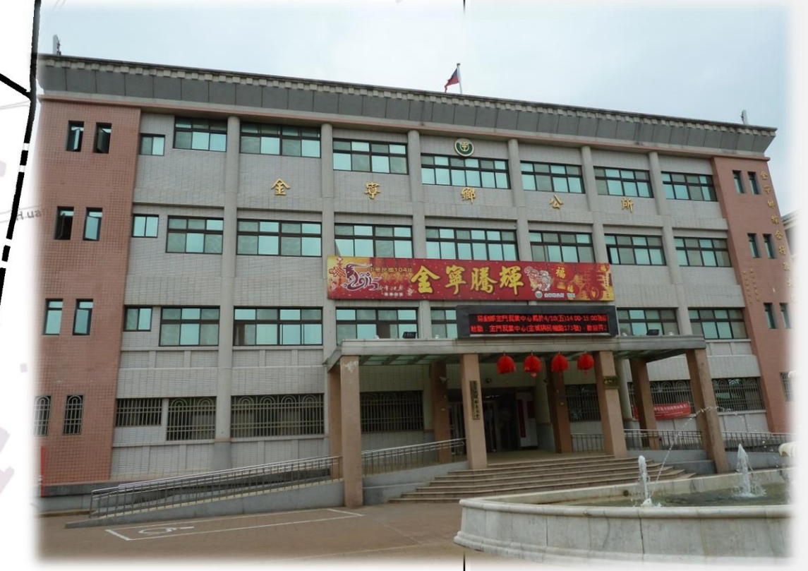
Jinning Township Administration Shelter for Flood, Earthand Tsunami
