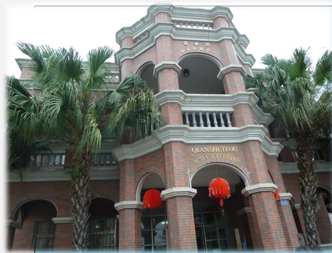
Qianshuitou Activity Center Shelter for Flood
