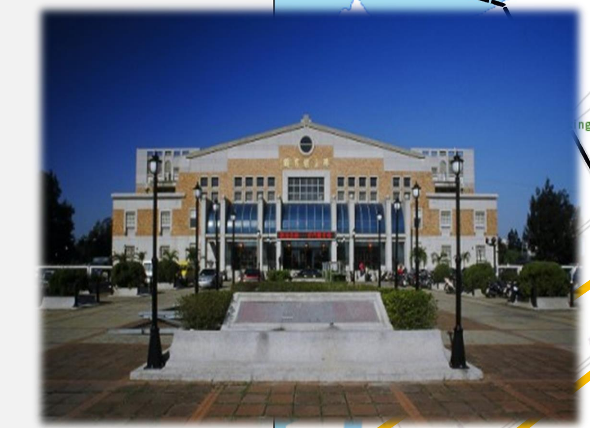
Kinmen Gymnasium Shelter for Flood
