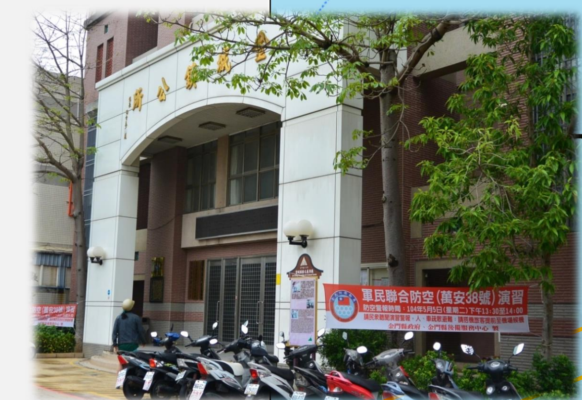
Jincheng Township Administration Shelter for Flood and Tsunami
