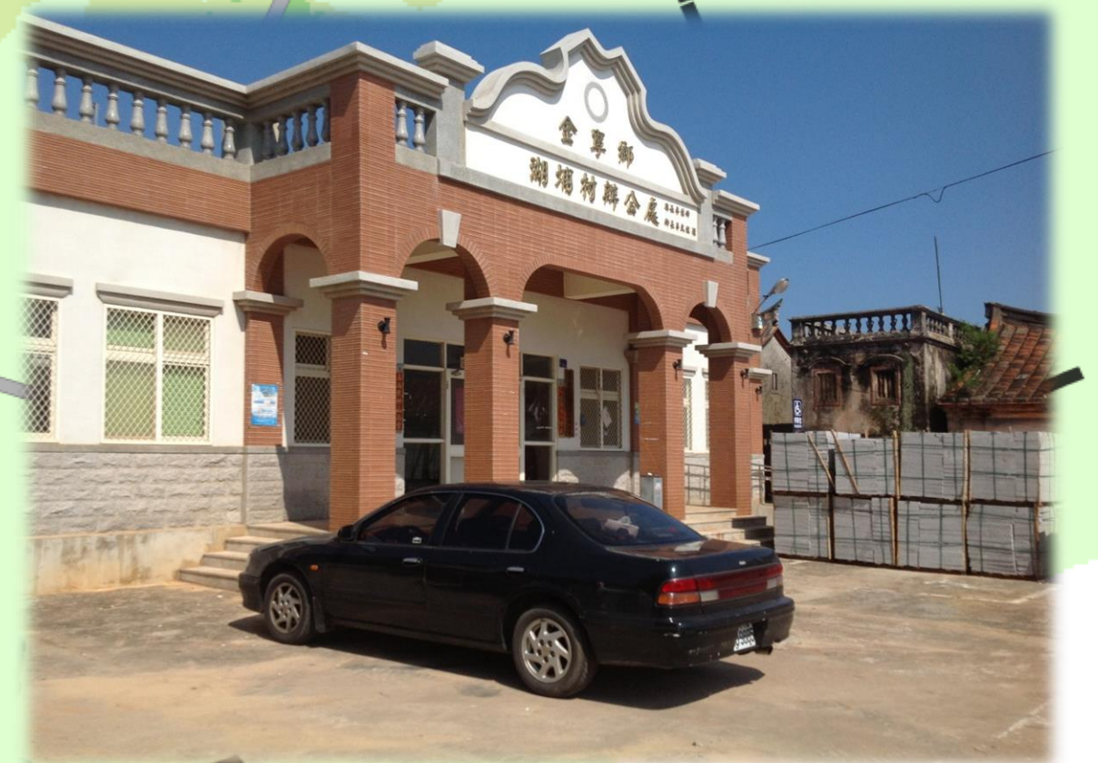
Banglin Village Office Shelter for Flood
